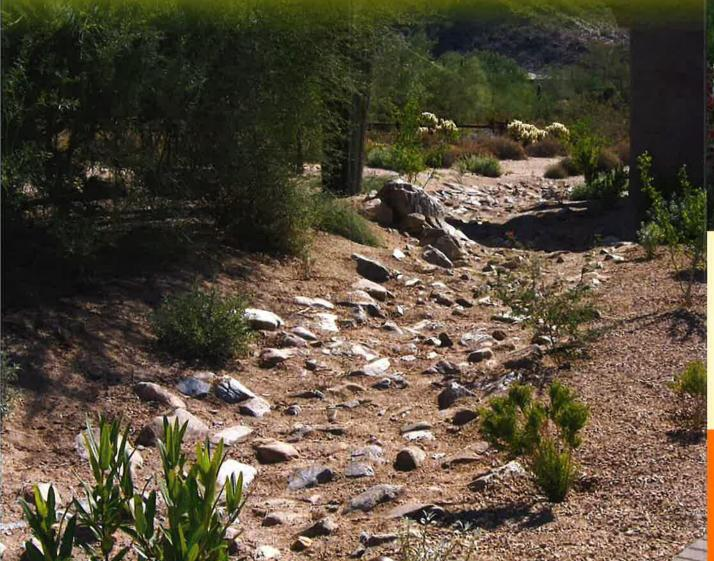
In the correctly constructed arroyo above, the large stones are fully integrated into the ground, and there is an incorporation of fine materials throughout. Also note that arroyos must be level within one inch, higher or lower, relative to the hardscape (pavers).
