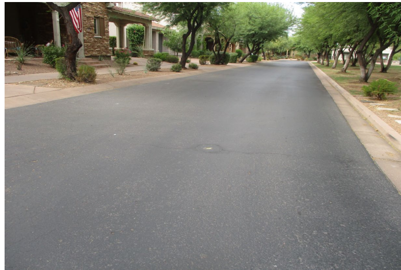
Terrace Homes West
