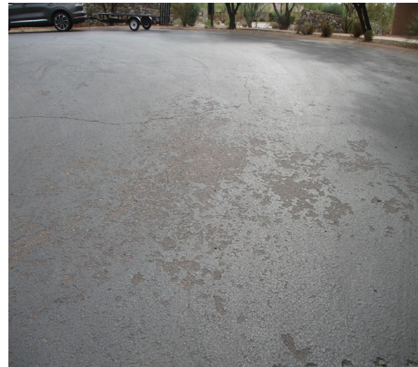
Terrace Homes West
